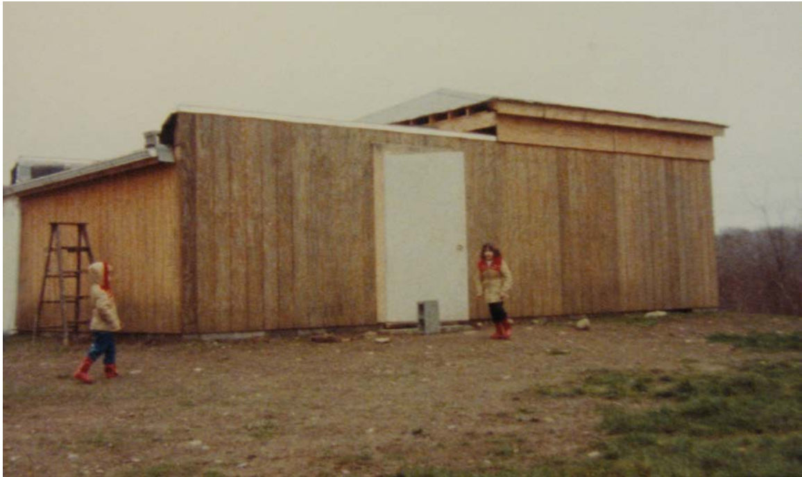
Indian Hill showing the observatory for the 16-inch just after it was completed.
